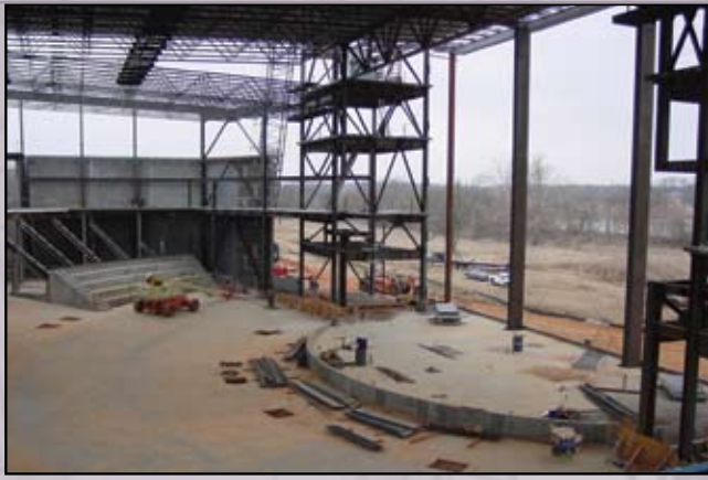
Construction on the Pinnacle Hills Worship Center's new sanctuary.
